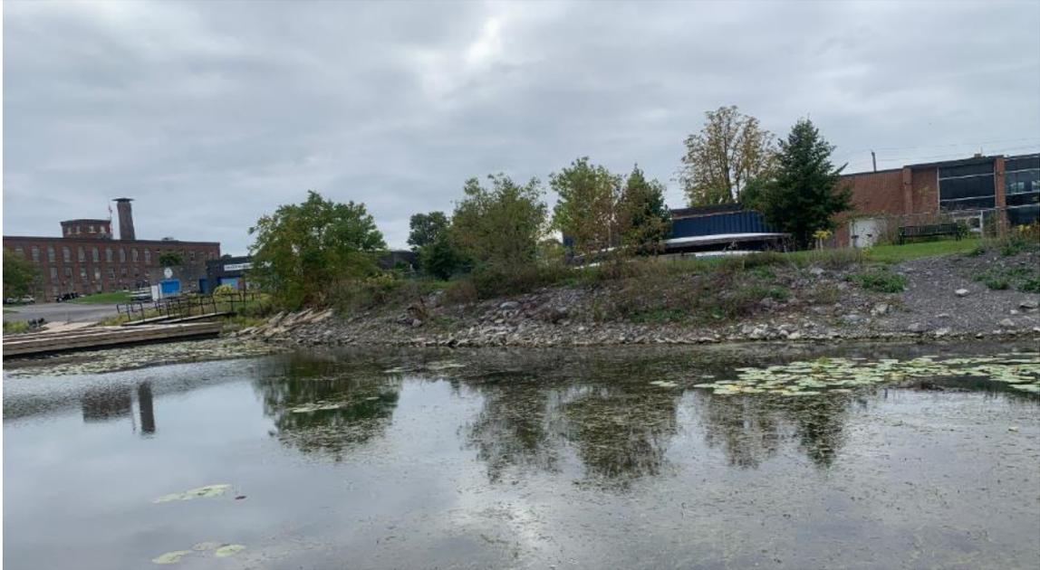
Existing rock armouring is present intermittently along the shoreline as bank protection. Typically consists of approximately 0.2 to 0.8 m diameter rocks on an approximately 6:1 slope.
