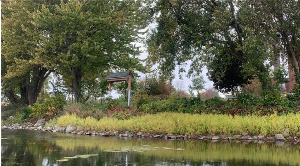
Existing rock armouring is present intermittently along the shoreline as bank protection. Typically consists of approximately 0.3 to 0.8 m diameter rocks on an approximately 10:1 slope.
